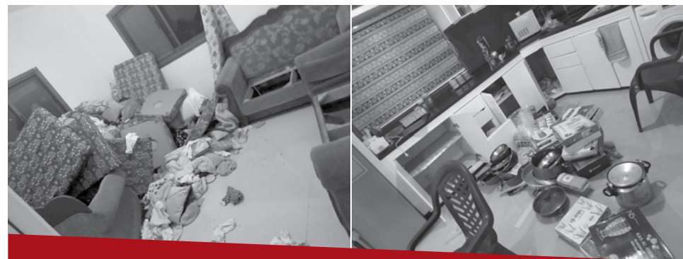
The destruction caused by the occupation forces to Hamayel family’s house in Beita
